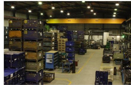
Before (400W High Pressure Sodium)
